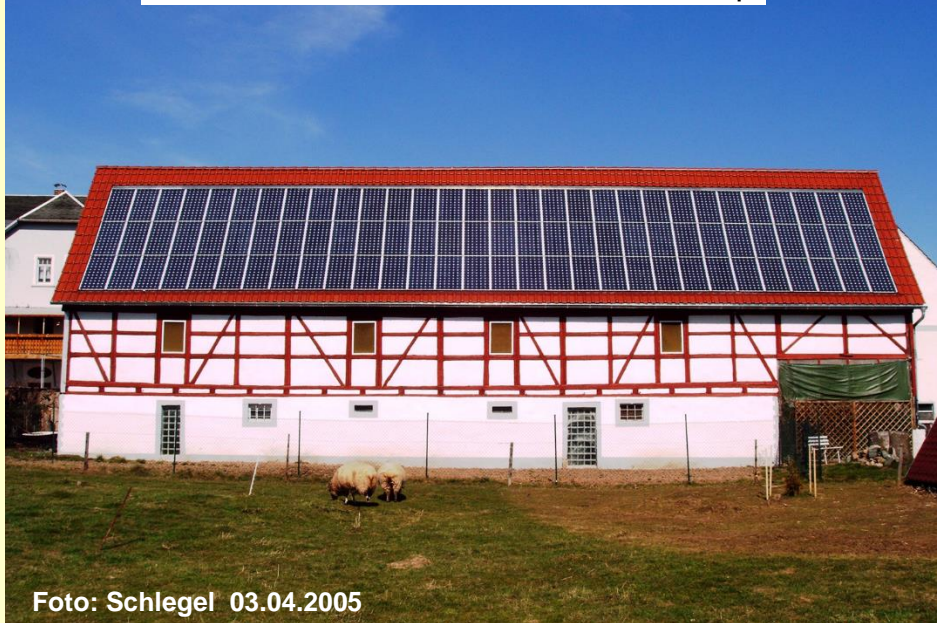
PV-Anlage Grunau (FG) - P = 15,75 \text{ kW}_p
